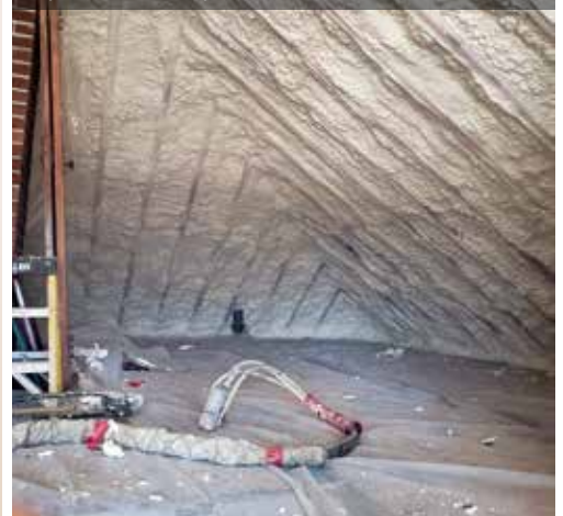
Spray foam helped with attic condensation.
